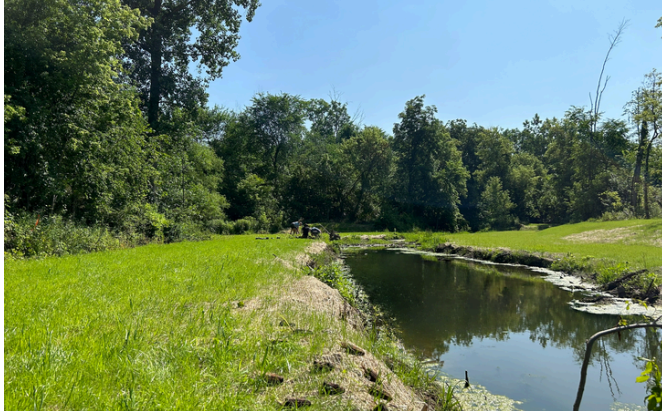
Completing the Floodplain Restoration Project at the Leisure Creek Condos
